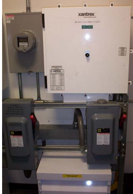
Figure 17: Final Inverter Installation
