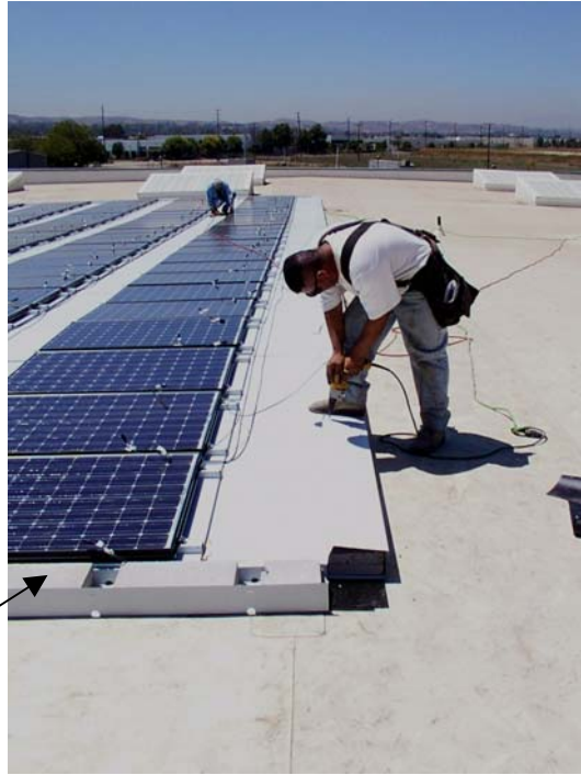
Figure 12: Installing perimeter ballasted curb
