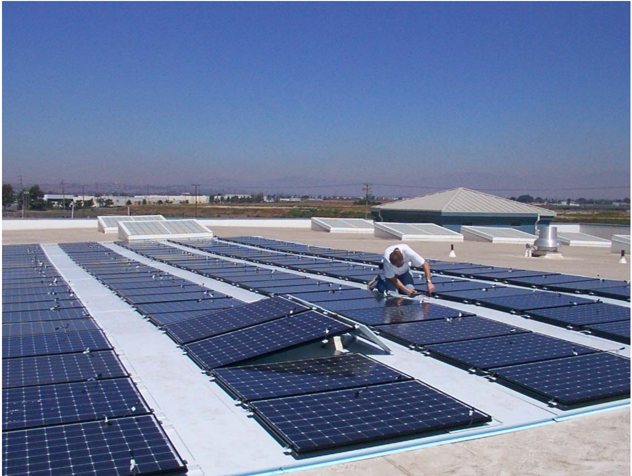
Figure 11: Installing grounding straps after all panels are placed on roof
