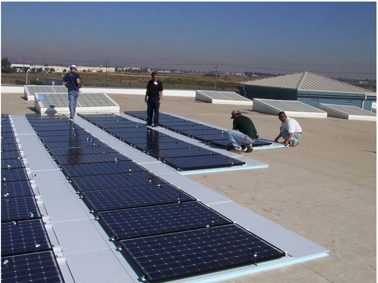
Figure 10 Interlocking panels with tongue-and-groove assembly
