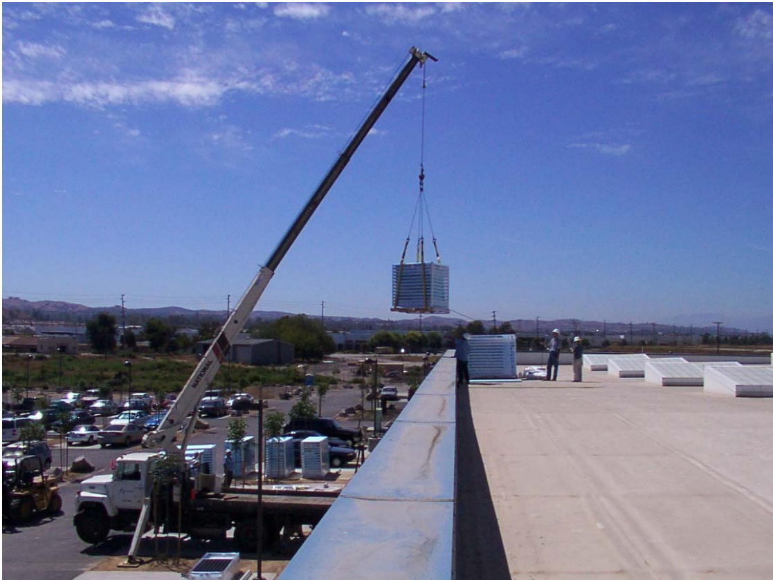
Figure 5: Shipping container being lifted by truck crane
