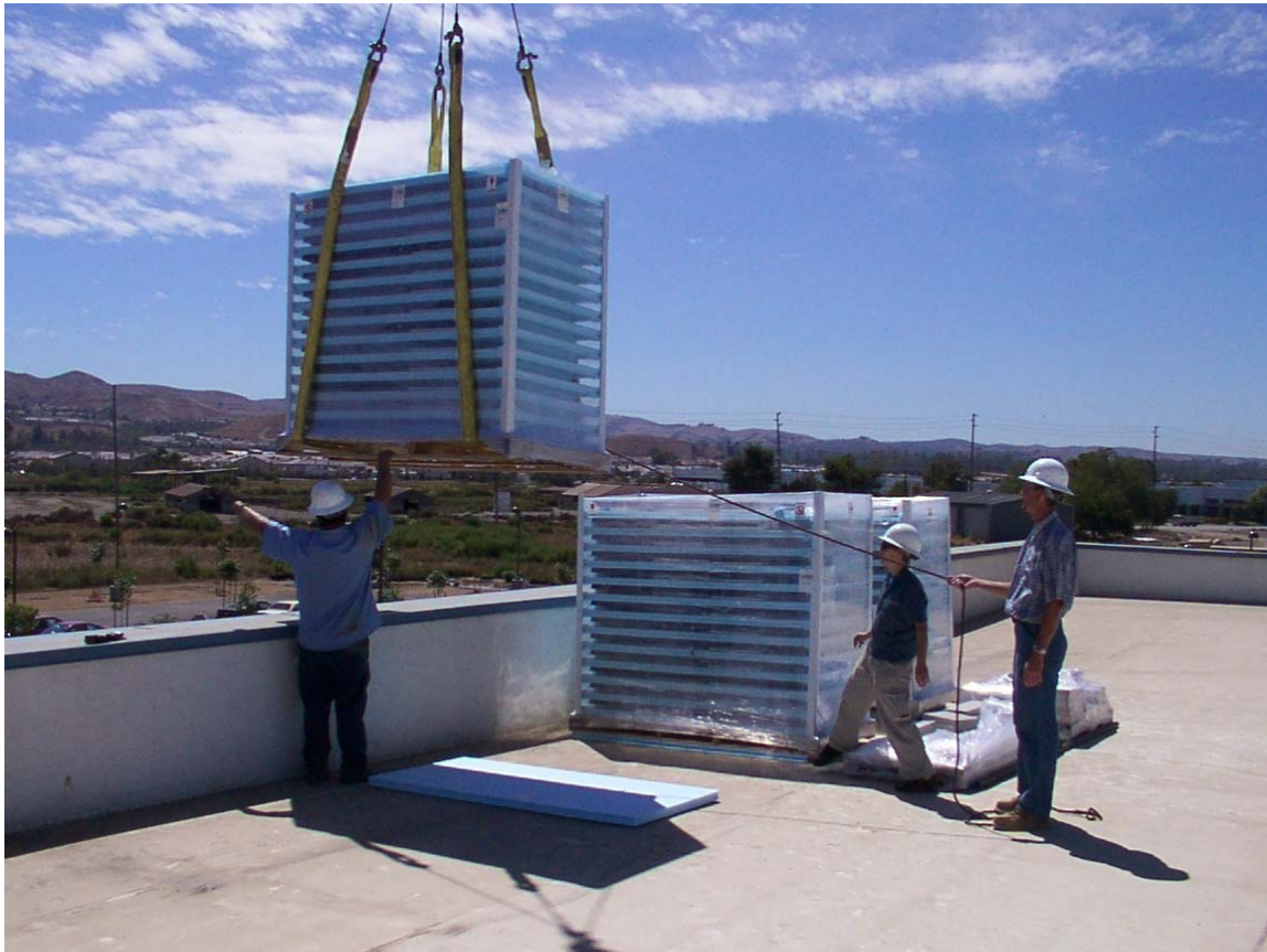
Figure 6: Setting panel pallet on polystyrene board to protect roof
